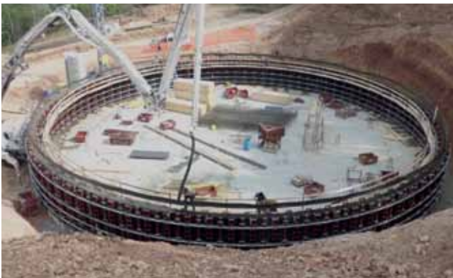
1 st concrete phase - H. 3,0 m
