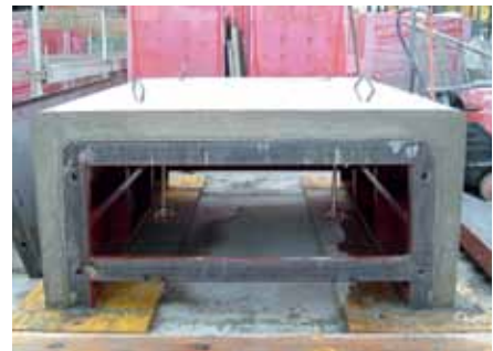
Whole casting of the prefabricated shaft
