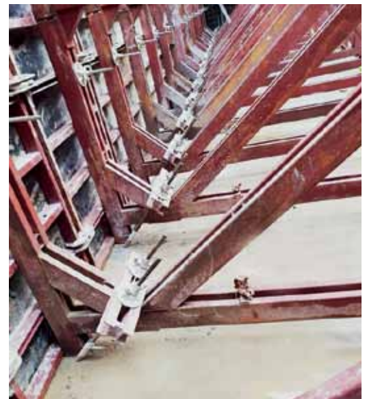
Example: Anchoring for side formwork, lost hexagon nut anchored in the foundation and in connection with recoverable tie rods and PVC tube.
