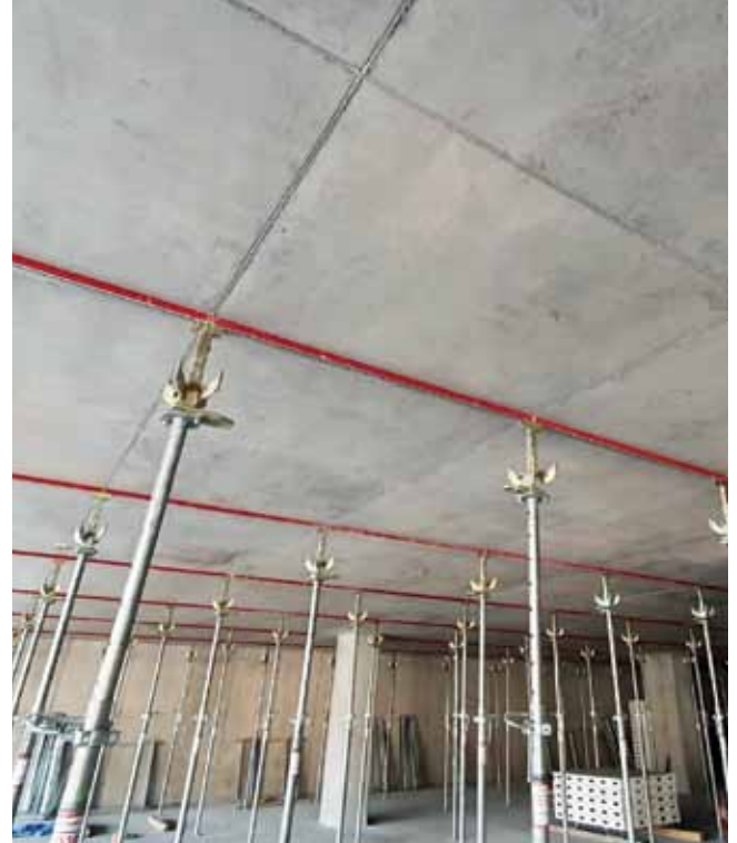
Early partial stripping of EVODECK elements
