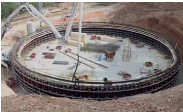
1 st concrete phase - H. 3,0 m
