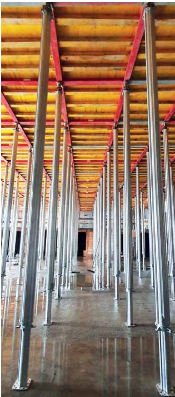
I-PROP ALU 625 Extension 480-625 cm Weight 31 kg
