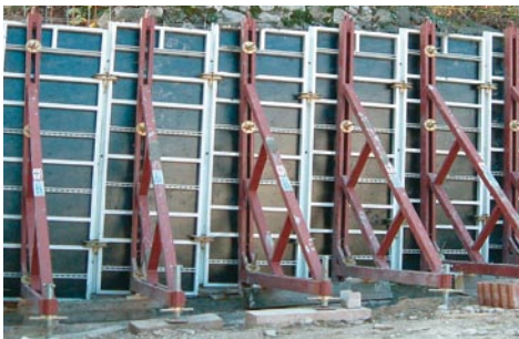
Supporting walls (single-sided forming)
