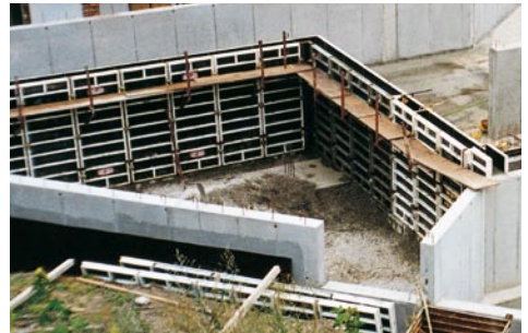
Corner formwork
