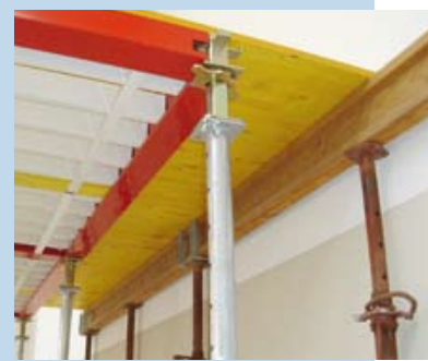
Intersection solution with traditional props
