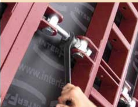
The elements are adjusted by means of a spindle in the radius (min. 3.0 meters)
